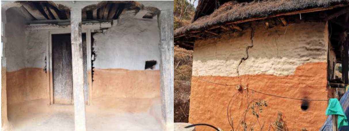
Figure 2: Examples of damaged houses after the Gorkha earthquake in 2015.
