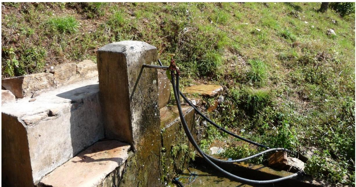
Figure 48: Leaking house water pipes connected to tap, Taluwa
